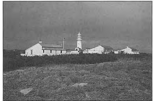
Plate 63. Lighthouse and associated buildings on Althorpe Island. Photo A. C. Robinson
