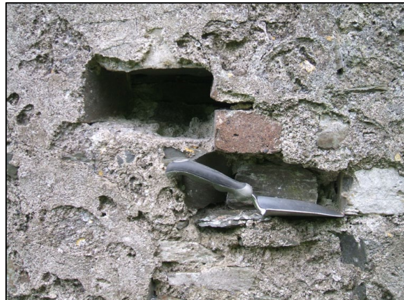
Top of chimney showing loose brickwork (left) and base showing mortar damage and loss of blocks (right).
