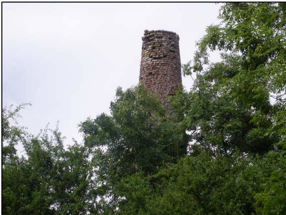
Top of chimney showing loose brickwork (left) and base showing mortar damage and loss of blocks (right).
