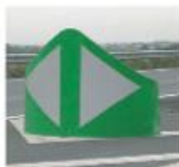
Figure 6.7: Nosing Marker Installation (France)
