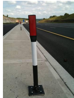
Figure 6.6: Delineator Post at a Layby
