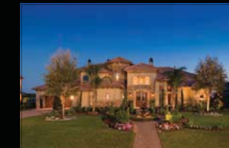
Houston's Best Custom Home Elevation: $1.8M - $2.5 Million Winner: Westport Homes, Inc. Finalist: Southampton Homes
