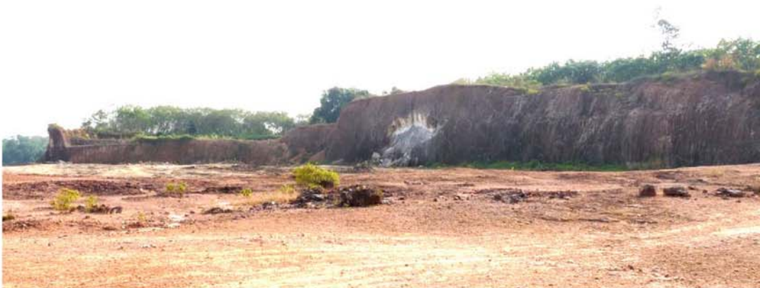
Fig. 10. Reclaimed area with part of the hill bulldozed
