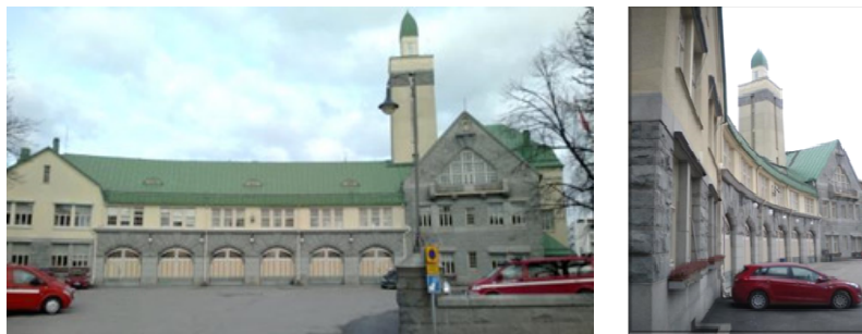
Picture 7. (left) The Tampere Fire Station with its granite walls (1908). [Photo by Sari Pommelin]
