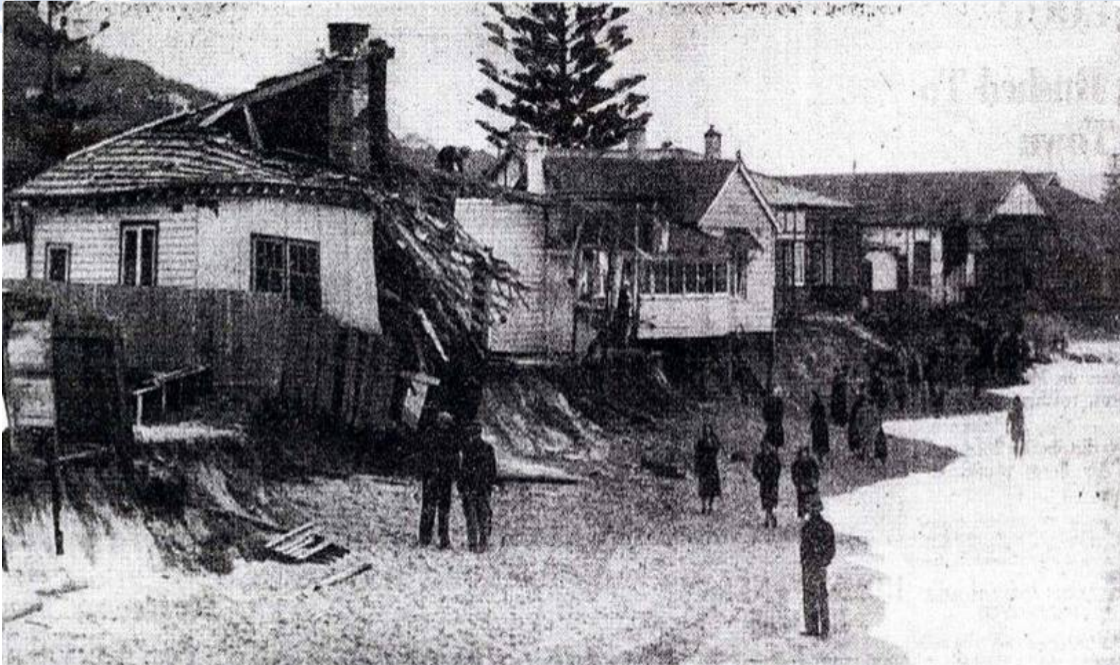
Damage to houses between Fielding St and Jenkins St, Collaroy. The Sydney Morning Auditor, 14.06.1945.
