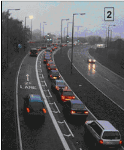
Figure 9 CCTV picture of new facility
