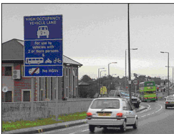
Figure 8 Illustration of the Leeds T2 Facility signage (source: Leeds University)
