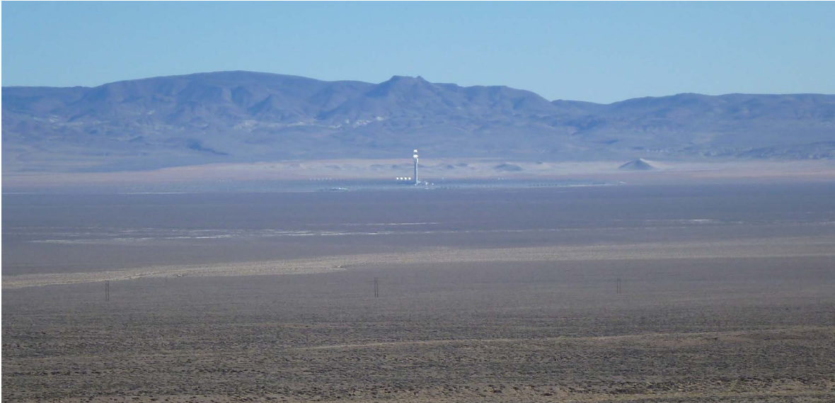
Photo 5.2 View from property of power lines and solar plant
