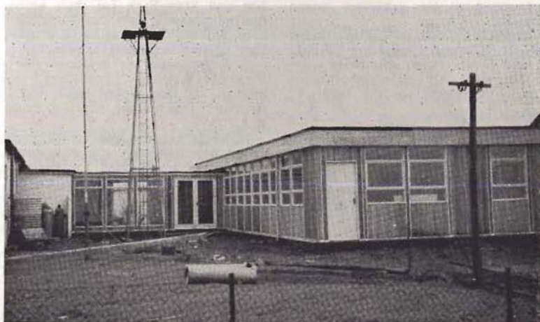
This new dormitory has replaced the Midland Gliding Club's old bunkhouse on the Long Mynd, 1,500 feet above sea level.
