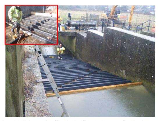
Figure 5: Baffle system from "Low Cost" modification of a crump weir at Jessop's Avenue, Bridport to improve fish passage"
