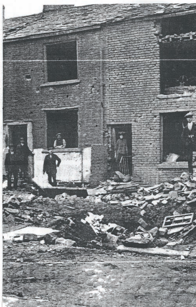
The Bolton raid. Bomb damage to the rear of houses in Kirk Street.
