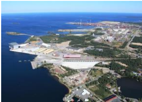
Figure. Kokkola – the area of hydrogen production with electrolyser, hydrogen pipes
