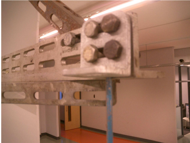
Figure 4.5: A detailed view of the clamped rod in the ground support
