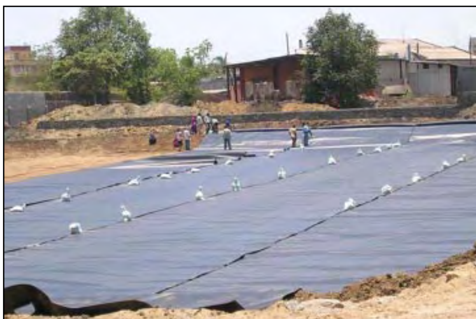
HW secured landfill work in progress at MIDC Tarapur
