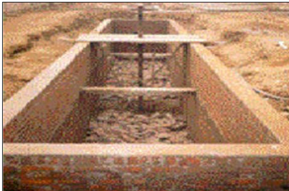
Rainwater harvesting structure at Nagpur
