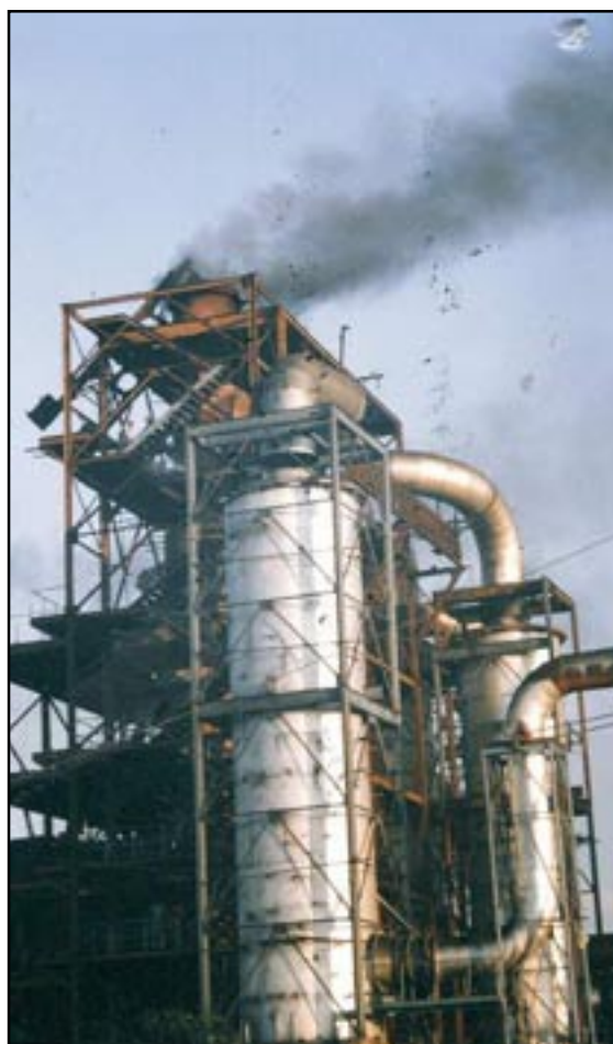
Problem sponge iron plant at Chandrapur
