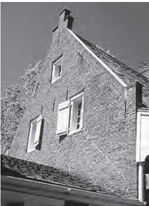
Figure 3 The south gable of the 1738 portion of the Lendeert Bronck house, Coxsackie, showing the vlechtingen (2002)
