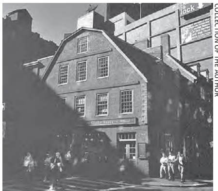
Figure 4 Building on the corner of Washington and School streets, Boston (2002)
