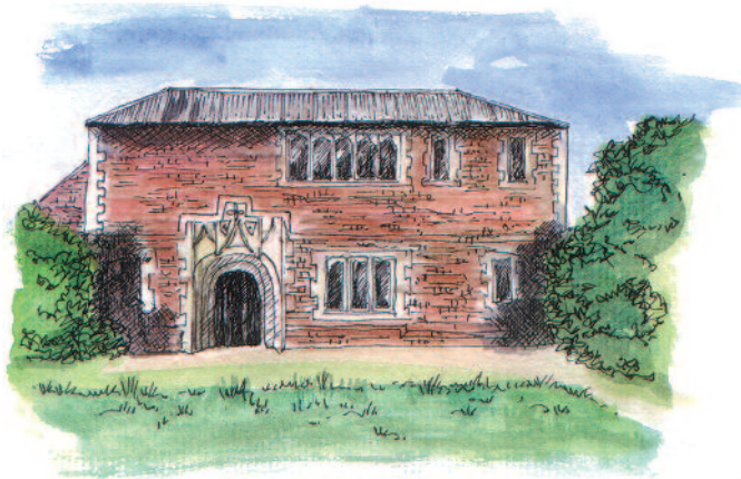
One of the two remaining portions of the fifteenth century palace, now part of Tower Farm in Little Downham
