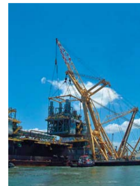
'Takilift 4' and 'Takilift 6' installing a module onto FPU 'P53'.
