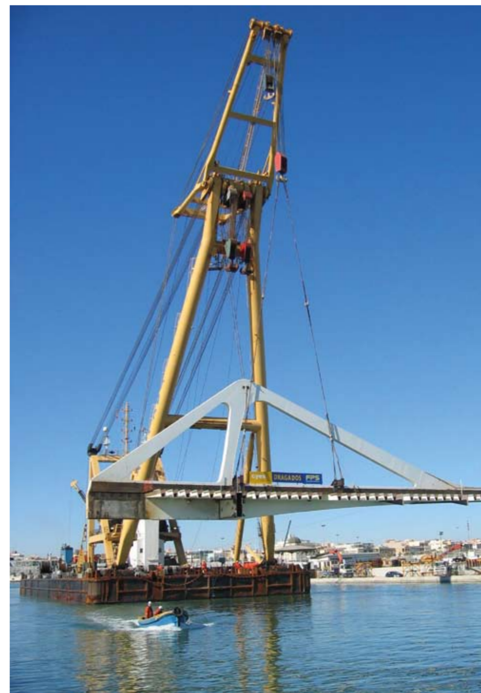
'Takilift 7' lifting a bridge section during the construction of a road bridge in Valencia.
