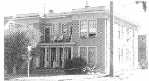
Buren/Holden Apartments 1908 708-10 So. 8th Street
