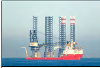
Pacific Orca Foundations Installation
