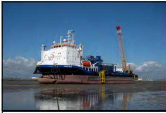
Stemat Spirit Laying Export Cables
