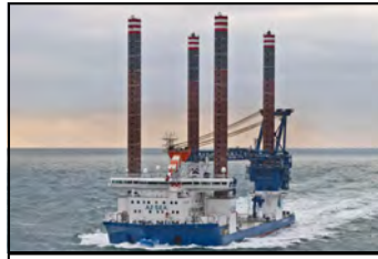
Sea Installer Turbine Installation
