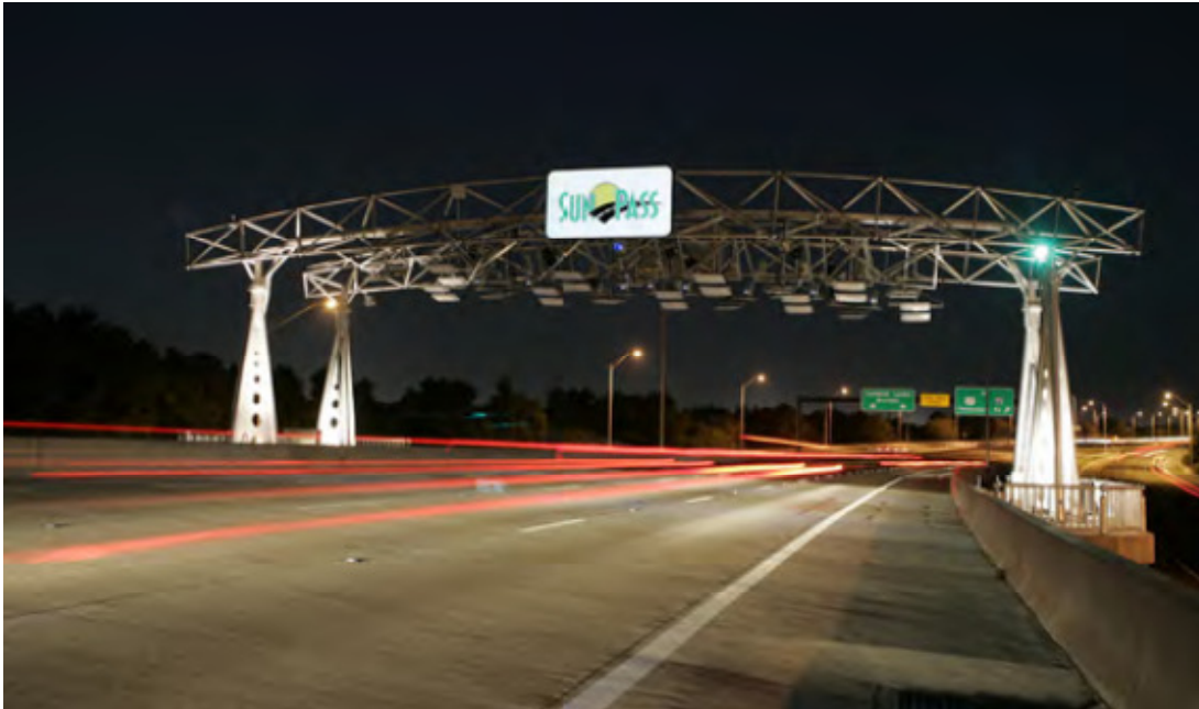
Figure 8: Florida's Turnpike Enterprise AETC Tolling Gantry
