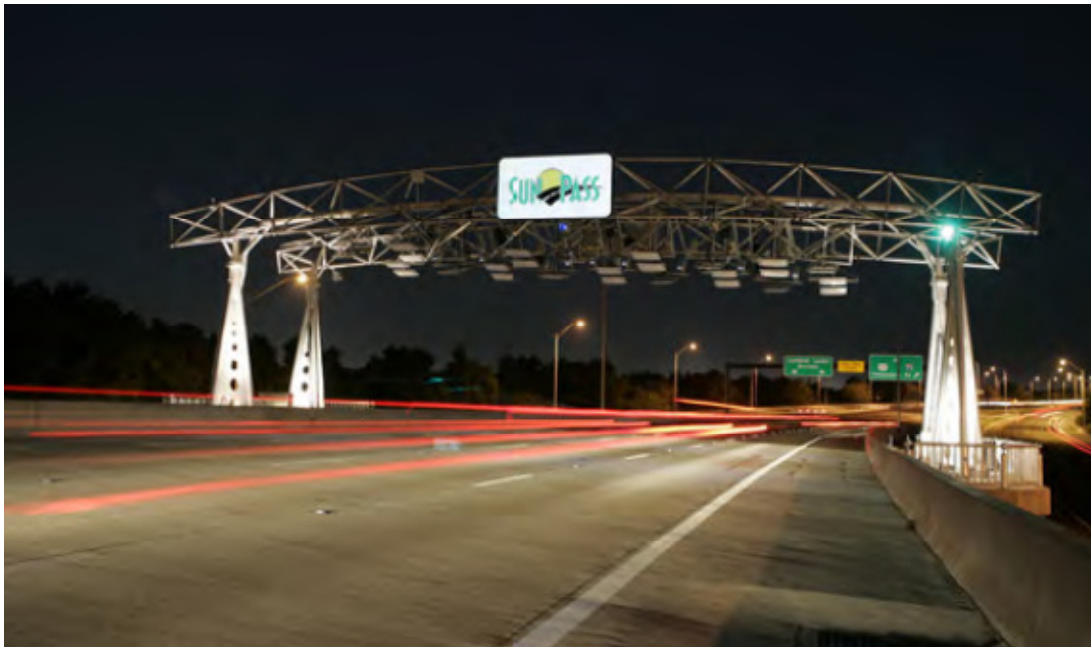
Figure 8. Florida's Turnpike Enterprise AETC Tolling Gantry
