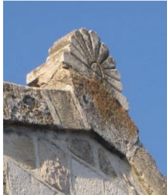
Crone on top of the roof
