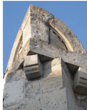
Corner of the roof
