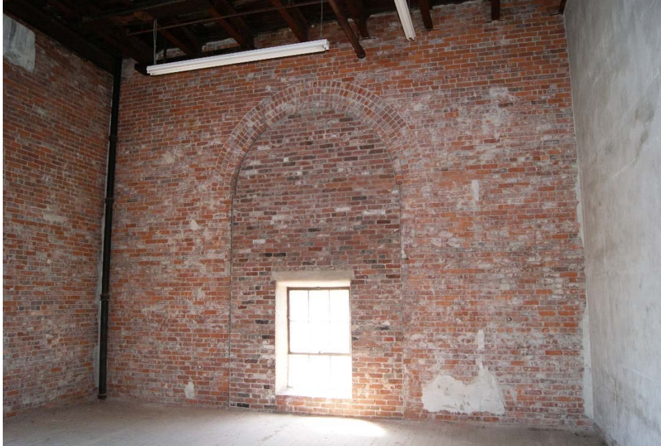
Photograph 5: American Brewing Company building, interior of Malt Mill core, room 301
