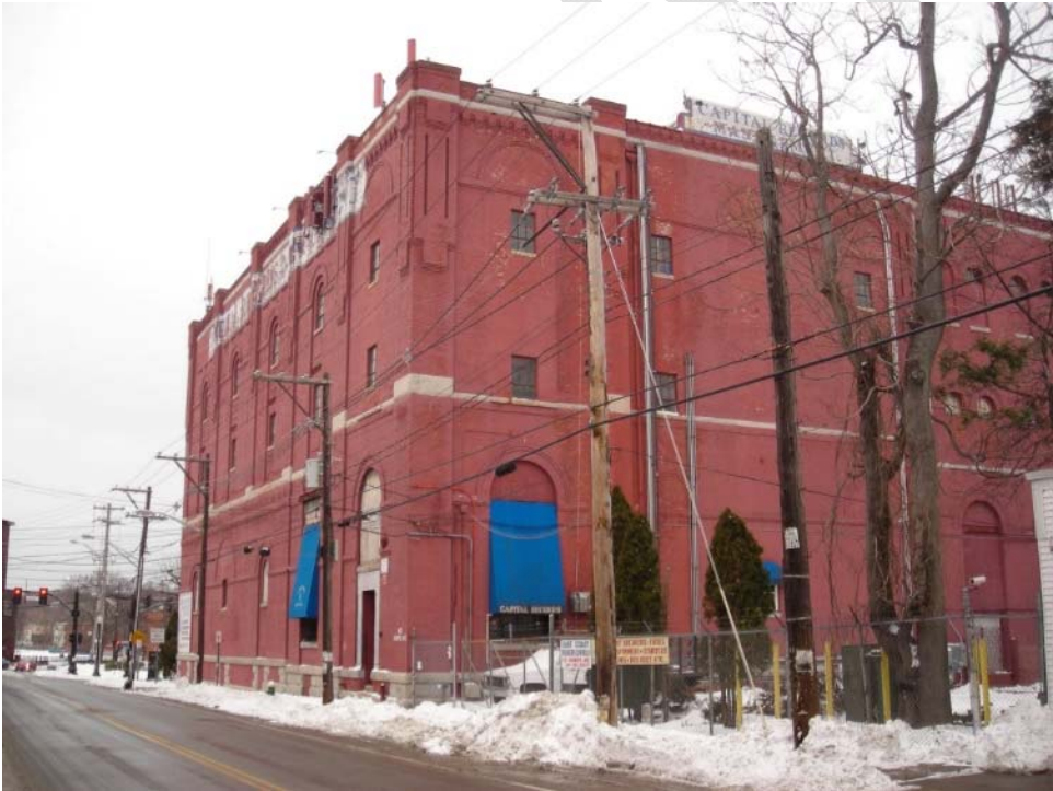
Photograph 2: View of American Brewing Company building, south and east elevations, facing west
