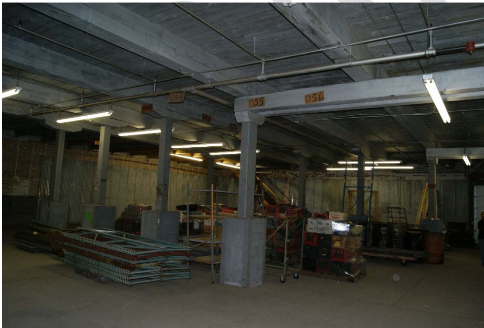
Photograph 12: American Brewing Company building, interior of Ice Plant, room 111
