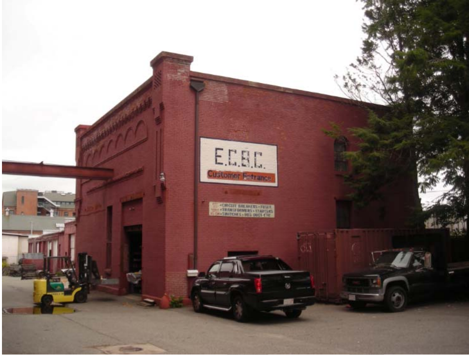
Photograph 13: American Brewing Company Second Boiler House, west and south elevations, view facing northeast
