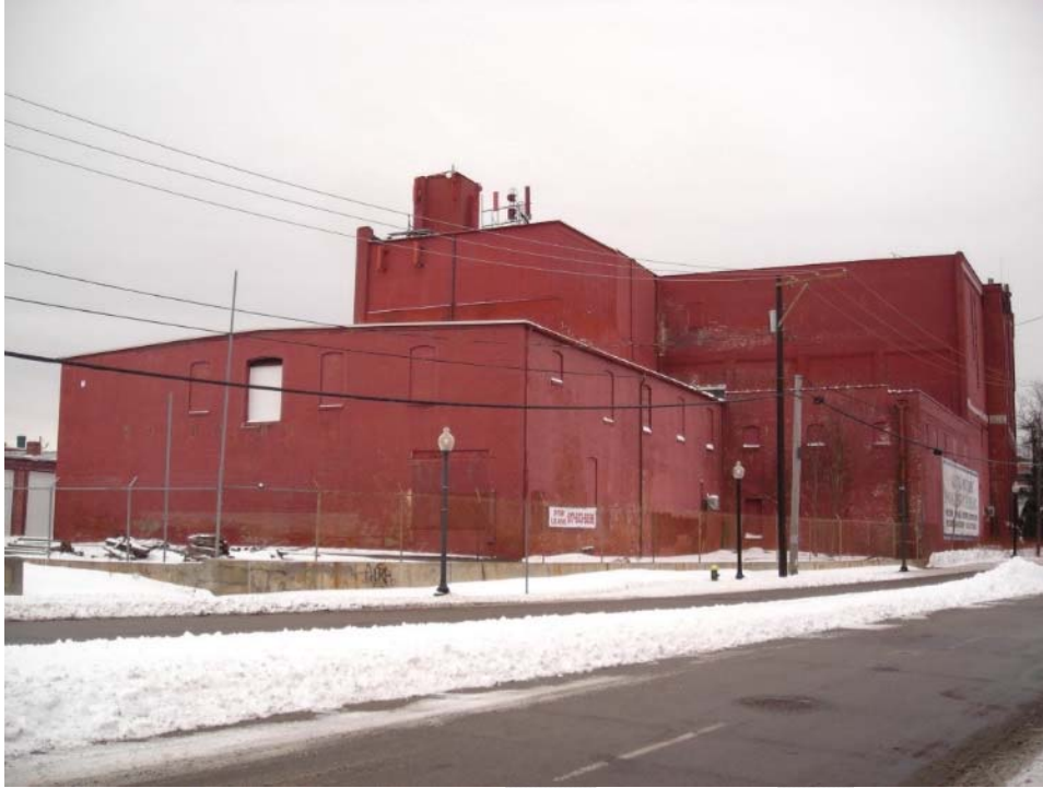
Photograph 3: View of American Brewing Company building, north and west elevations, facing southeast
