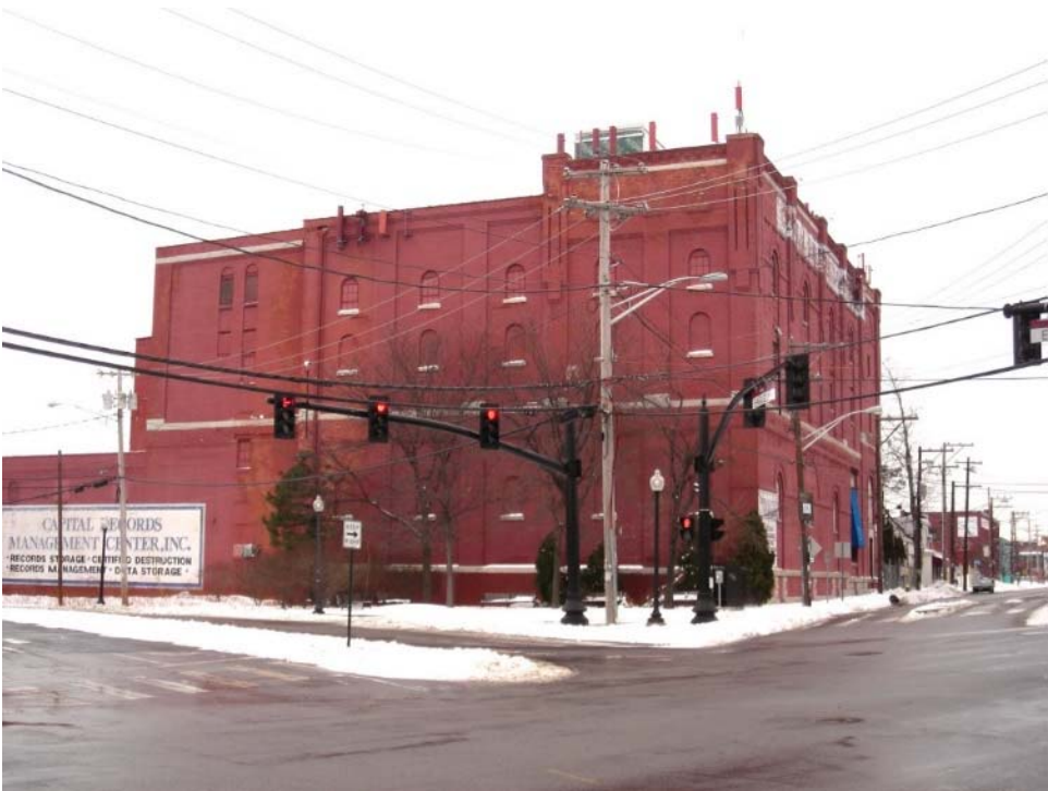
Photograph 1: View of American Brewing Company building, west elevation, facing east
