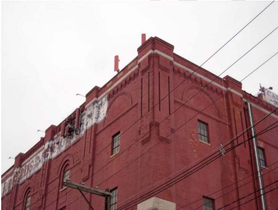
Photograph 4: Detail of southeast corner of American Brewing Company building, facing northwest
