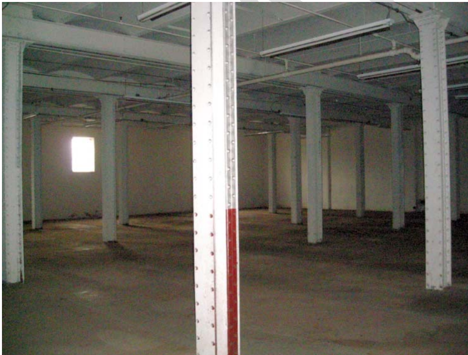
Photograph 8: American Brewing Company building, interior of Stock House core, room 204 (Fermenting).
