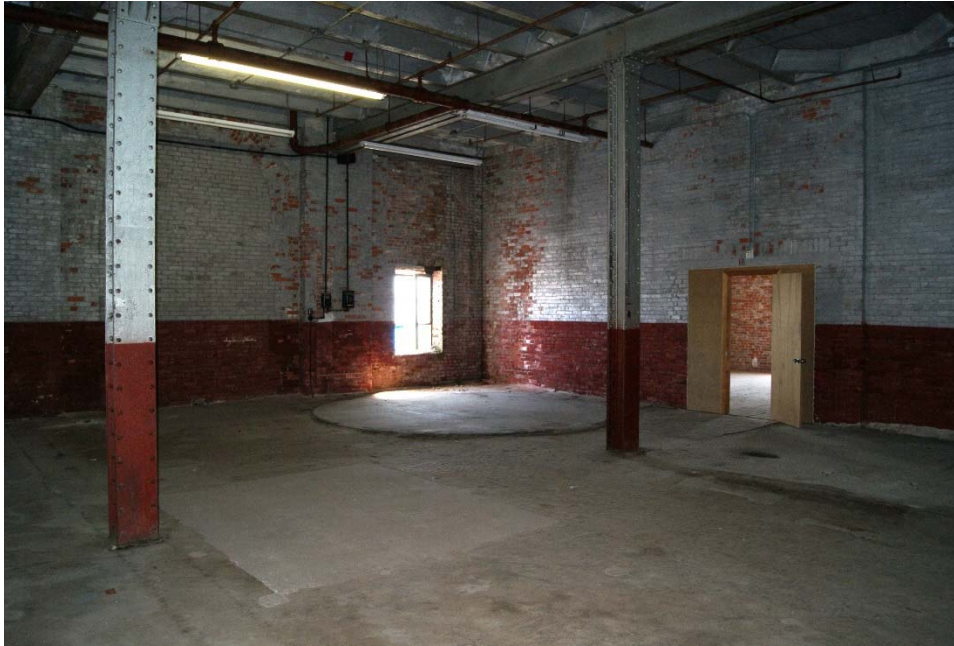
Photograph 7: American Brewing Company building, interior of Brew House core, room 302. Note floor patches.
