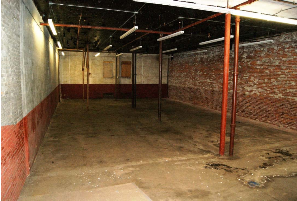
Photograph 9: American Brewing Company building, interior of Lager Racking core, room 306
