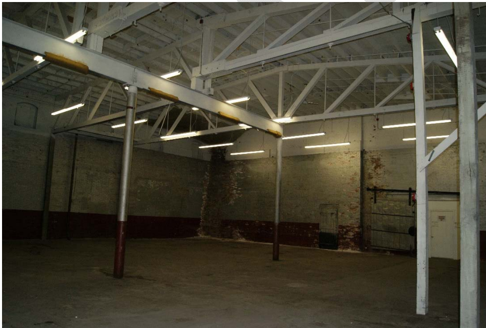
Photograph 10: American Brewing Company building, interior of Lager Wash House, room 109
