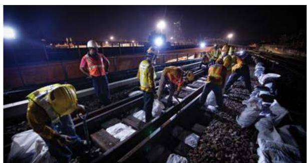
Replacing 96,000 sleepers on the NSL while the city slept.
