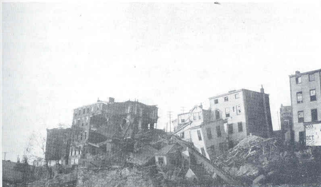
BUILDING COLLAPSING AS THE SIDE HILL SLIPS The steep side hills are often treacherous for buildings
