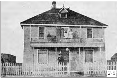
Strathcona Cottage Hospital, 1906
