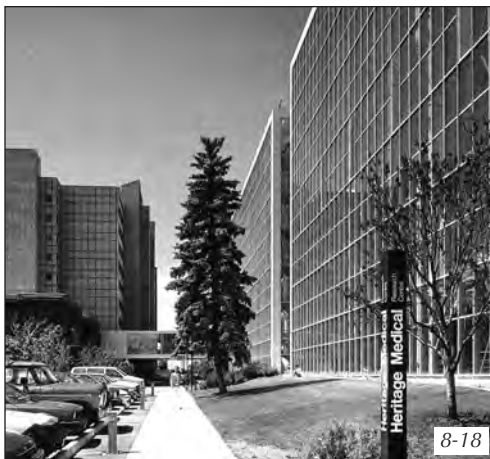
First HMRC research buildings 1984-88
