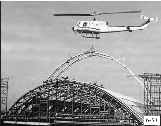
Placing the glass top on the WCM HSC, circa 1980
