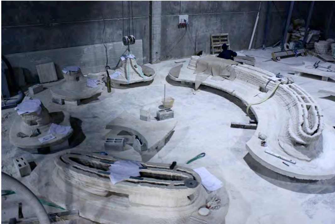
Figure 23 - Full scale Radiolaria under construction (image courtesy of Enrico Dini)
