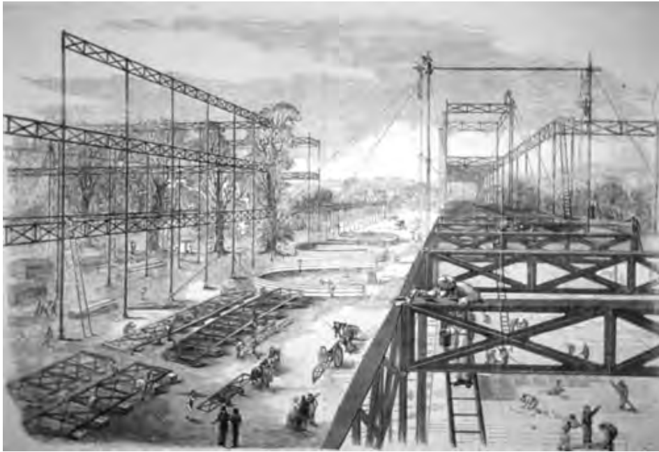
Figure 64 - Joseph Paxton's Crystal Palace. Drawing of the assembly of industrialised components. Image source - http://ww3.barrington220.org/bhs/fine_arts_folder/AStevenson/Interrelated_Arts/EngineeringArchitecture.htm Access date 25th August 2011
