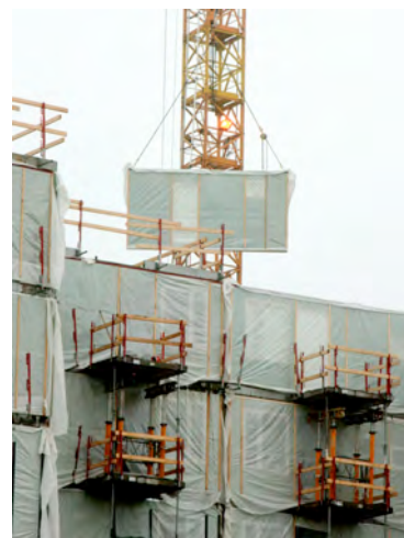
Figure 69 - Skanska Precast concrete panel factory in Stragnas, Sweden. Composite panels of timber and plasterboard being lifted into place on site in Stockholm, Sweden. Photos by James Gardiner
