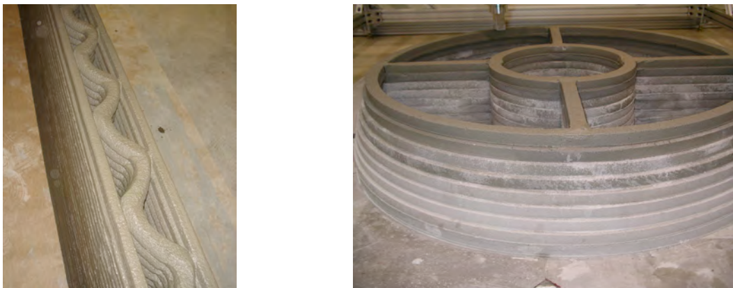
Figure 15 (a) Contour crafting - wall test (b) Contour crafting - Scaled down adobe structure test - Both images courtesy of Dr Khoshnevis, USC)
