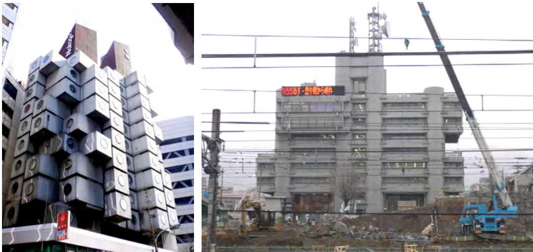
Figure 74 – Nagakin Capsule Tower in Ginza by Kisho Kurokawa 1970. Yamanshi Press building 1967 in Kofu by Kenzo Tange. Photos James Gardiner 2006
