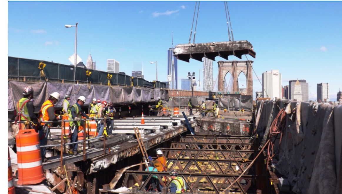
Work crews perform operations at the York Street Structure above the BQE. The roadway deck was fully removed to allow for full replacement of the underlying structure.
