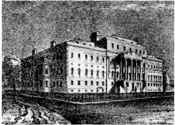
50. Marine Hospital, Quebec City, Quebec
