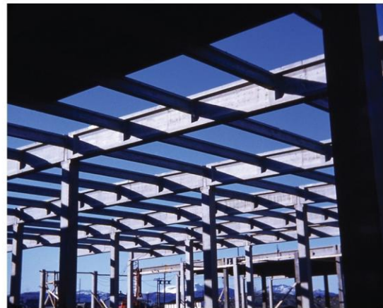
"Membership Certificate" – Architect-Engineers, Narsarssuak, Greenland Muskegon Indian steel fabricators on the Radio Tower, Narsarssuak Schokbeton building system, under construction, Narsarssuak
