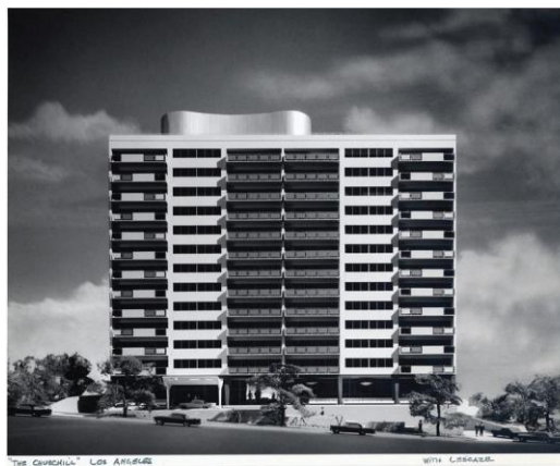
Ken Snelson's 'Structure' on the way to the New York Worlds' Fair, 1964 The Colombian Center, Federacion National de Cafeteros de Colombia, New York, 1966 The Churchill Apartments, Wilshire Boulevard, Los Angeles, with William Lescaze, 1969
