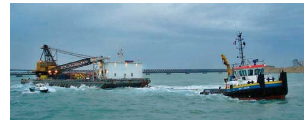
'Smit Bison' transported the crane barge 'Missing Link' towards the 'Rokia Delmas' casualty location.
