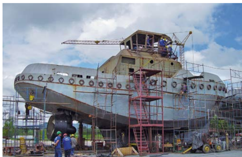
The first newbuildings for SMIT Rebras under construction at the Detroit yard at Santa Catarina.
