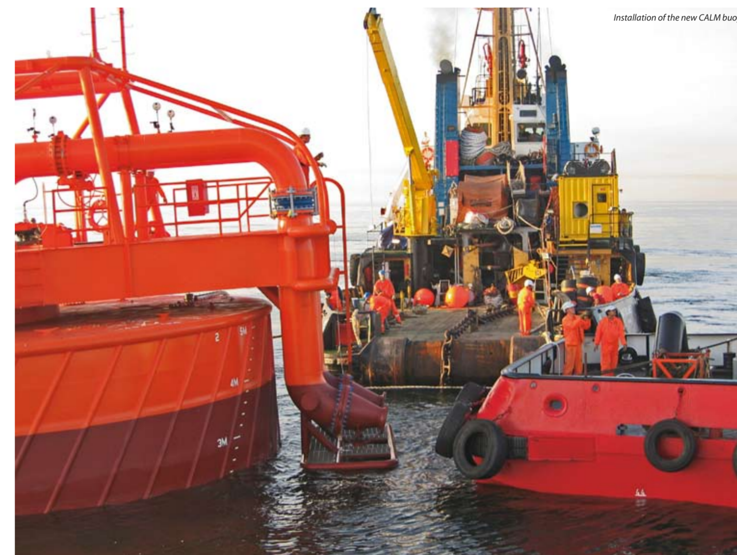
Installation of the new CALM buoy.
