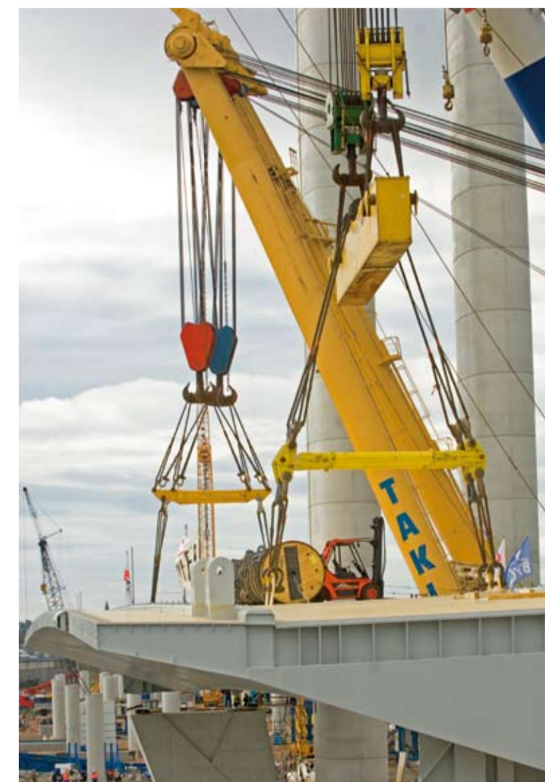
'Taklift 7' and 'Matador 3' install the second bridge section in a dual lift.
