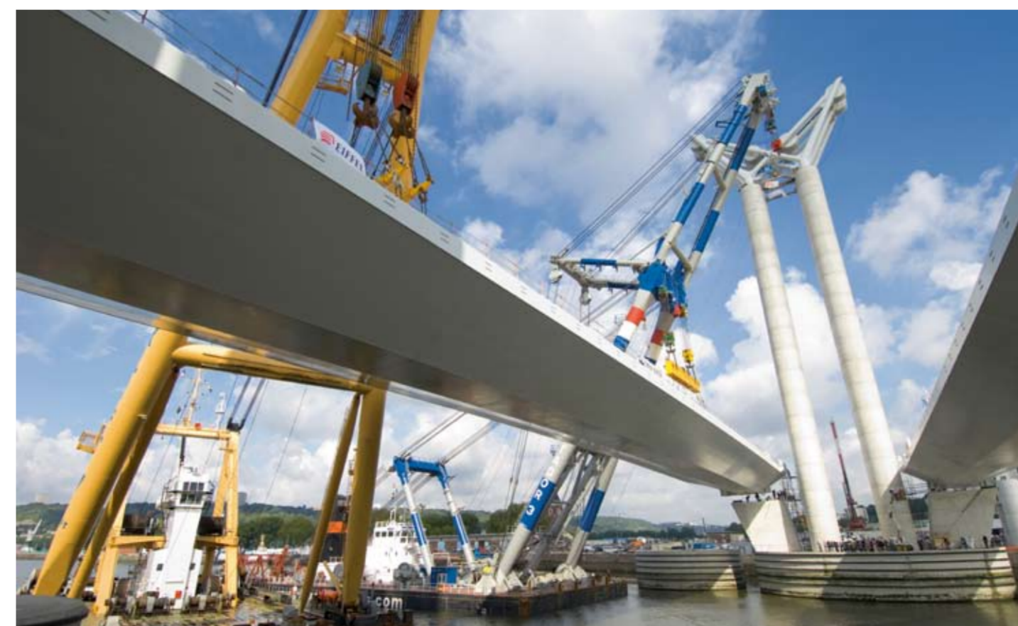
'Taklift 7' and 'Matador 3' install the second bridge section in a dual lift.
