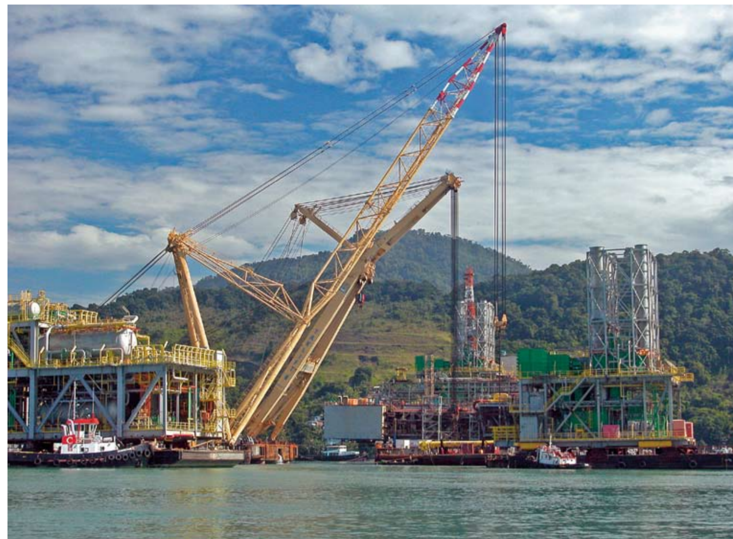
Sheerlegs 'Taklift 4' and 'Taklift 7' installing the modules on FPSO 'PS2', in Brazil.
