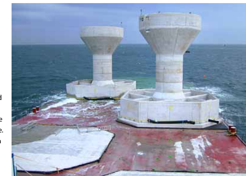
Turbine foundations on the deck of the 'Giant 4'.
