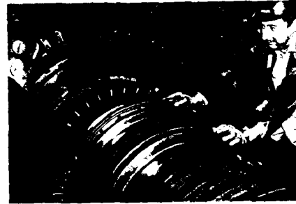
Exhibit III-C. When station service was lost at the Ravenswood plant of Consolidated Edison, oil pressure circulation to the bearings of the 1,000,000 Kilowatt Unit No. 3 was lost. The machine was taken off the line, but the bearings were damaged and the journal, shown above, was scored during the run-down period.
