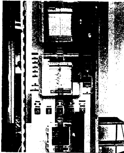
Exhibit I-R. These recording meters, at the Syracuse Area Control Center of Niagara Mohawk Power Corporation, give the system operators an
