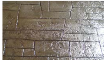
STYLE: Old World Cobblestone PRODUCT USED: H&C Dry Shake Color Hardener H&C Dry Shake Color Release H&C Low VOC Concrete Sealer Clear Gloss Oil COLORS FEATURED: Tweed (Color Hardener) Bold Bark (Color Release)
