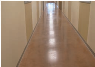
STYLE: 200-Grit Honed Finish PRODUCT USED: H&C Acetone Dye Stain H&C Clear Liquid Hardener & Densifier H&C Lithium Protective Finish COLORS FEATURED: Desert Orange (Acetone Dye) Vegas Light (Acetone Dye)
