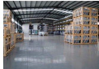
STYLE: 800-Grit Semi-Polished Finish PRODUCT USED: H&C Clear Liquid Hardener & Densifier H&C Lithium Protective Finish COLORS FEATURED: None Clear Finish
