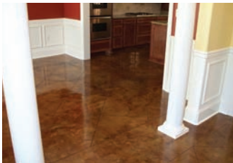
STYLE: 800-Grit Semi-Polished Finish PRODUCT USED: H&C Acetone Dye Stain H&C Clear Liquid Hardener & Densifier H&C Lithium Protective Finish COLORS FEATURED: Saddle Brown (Acetone Dye) Reno Gold (Acetone Dye)
