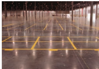
STYLE: 1500-Grit Highly Polished Finish PRODUCT USED: H&C Clear Liquid Hardener & Densifier H&C Lithium Protective Finish COLORS FEATURED: Spanish Dagger (Acetone Dye)
