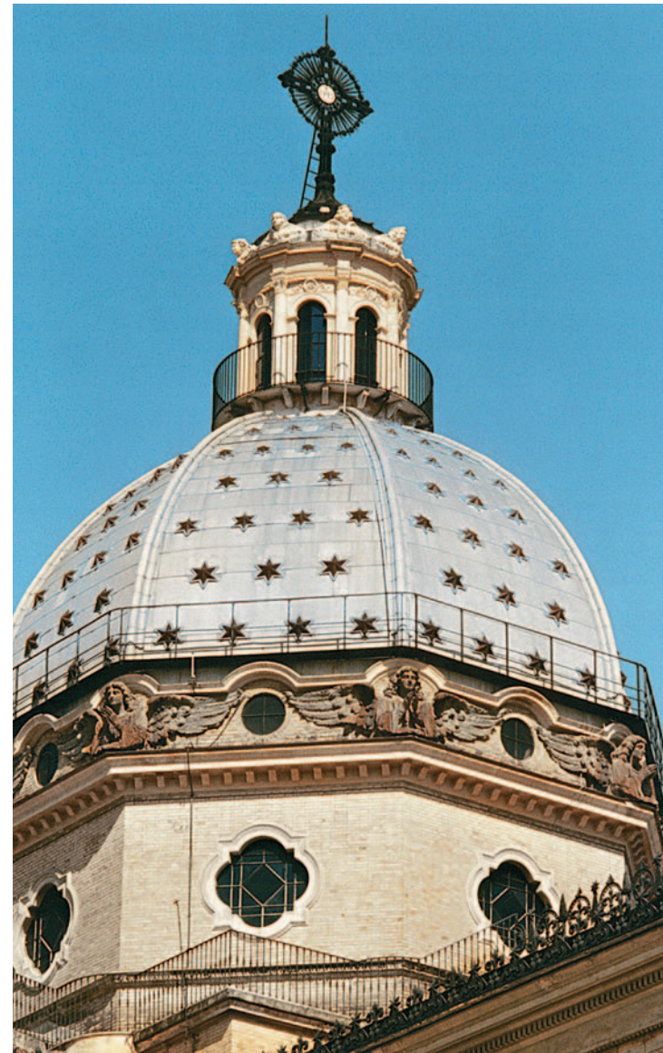
Raffaele Ingami. San Gioacchino in Rome, 1890s (the dome is lined with aluminium)
