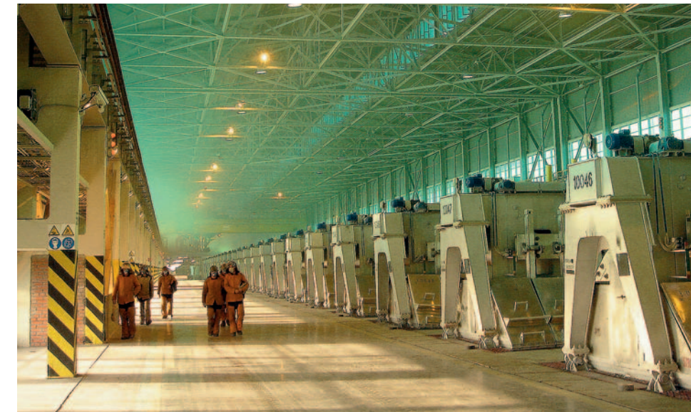
Reduction area at a modern aluminium smelter (Khakas Aluminium Smelter)
