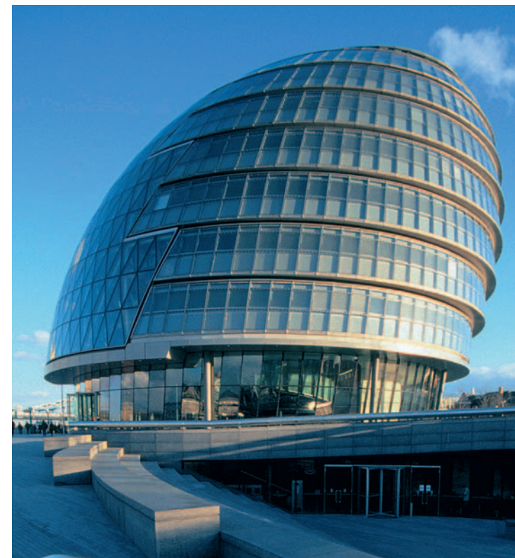
Norman Foster. City Hall (London), 2003 (lining is made of glass-covered aluminium panels)
