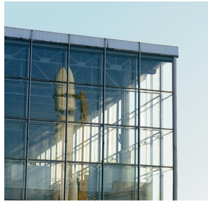
B.S. Vilensky et. al. Chemical Industry Pavilion at VDNKh (VVTs), Moscow, 1976 (the house frame is made of aluminium)
