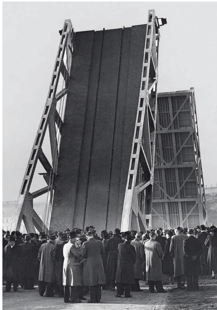
Drawbridge made of aluminium in Sanderland, UK, 1950
