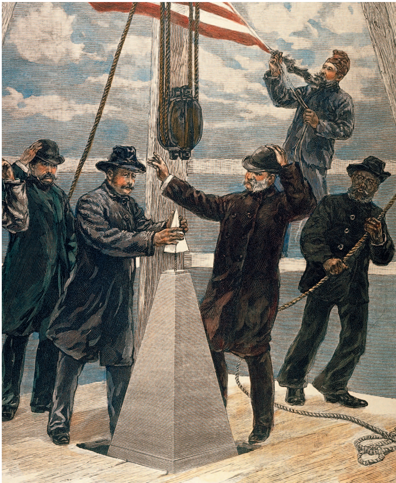
Mounting the aluminium capstone on the Washington Monument. Copperplate after a drawing by S. Nealey, 1884
