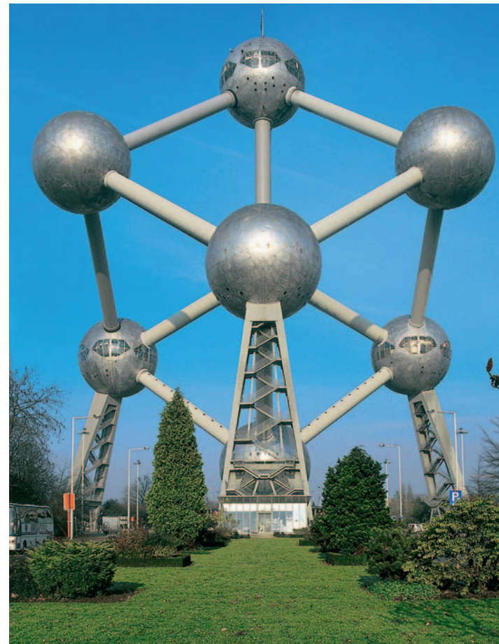
André Vaterceyn. Architectural monument Atomium, Brussels, 1958. Reconstruction, 2006 (spheres are covered with aluminium plates)
