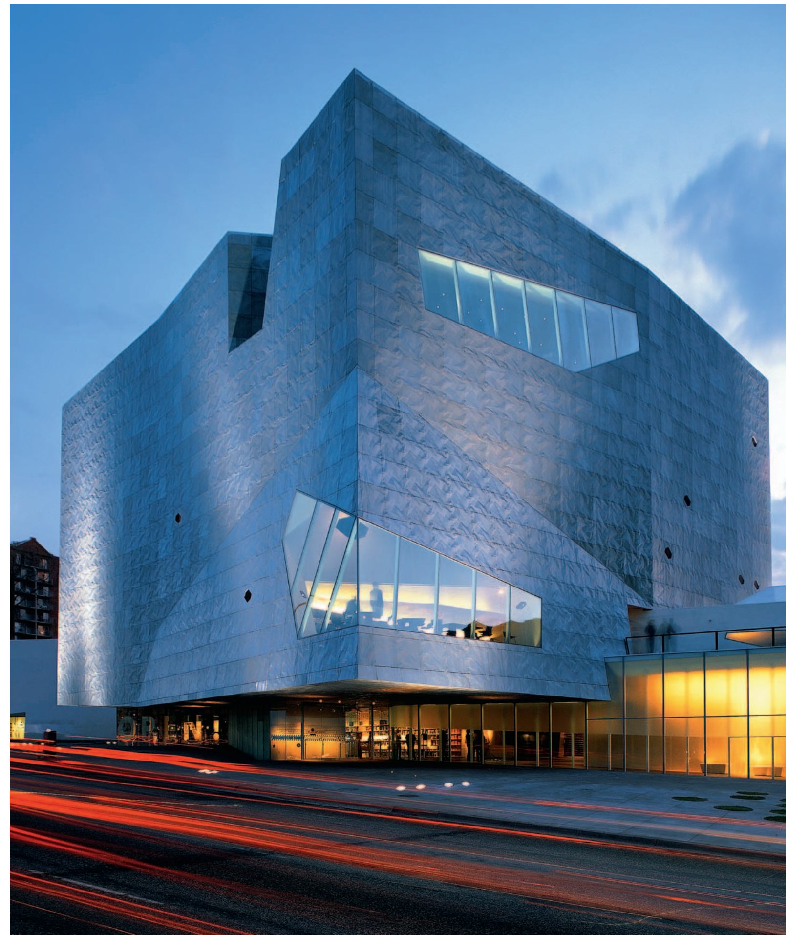
Jacque Herzog, Pierre de Meuron. Walker Art Center in Minneapolis, USA, 2005 (the building's lining is made of aluminium)
