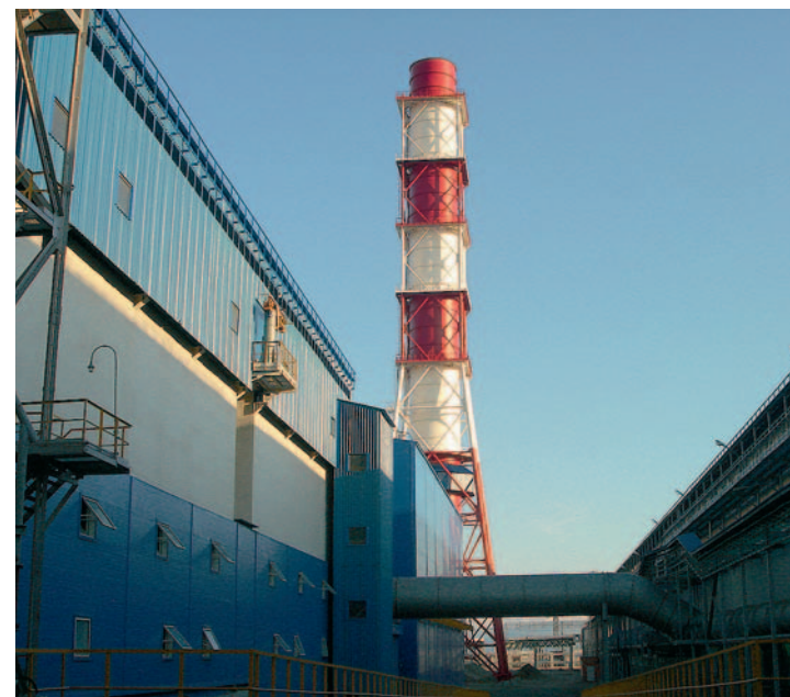
Exhaust gases' cleansing block at Khakas Aluminium Smelter
