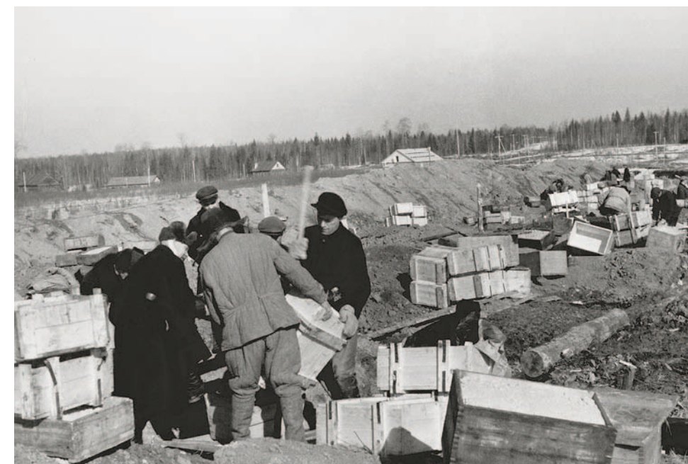
Laying explosives in demolition shafts at Tikhvinsky bauxite mines, 1936
