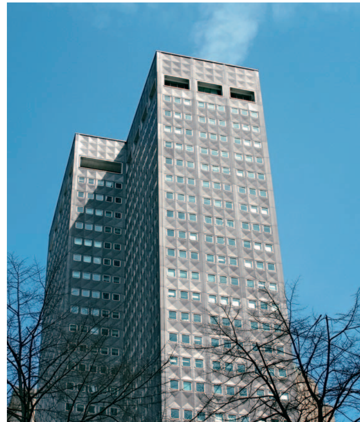
Harrison & Abramovitz. Alcoa Building, Pittsburg, 1950–1953 (the building's walls are made of aluminium panels)
