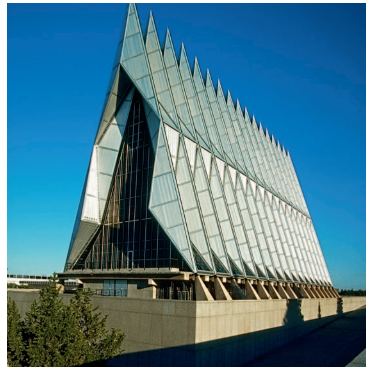
Walter Netsch, Jr. (Skidmore, Owings & Merrill). Cadet Chapel at the U.S. Air Force Academy in Colorado Springs, 1956–1962 (the building's walls are made of aluminium panels)
