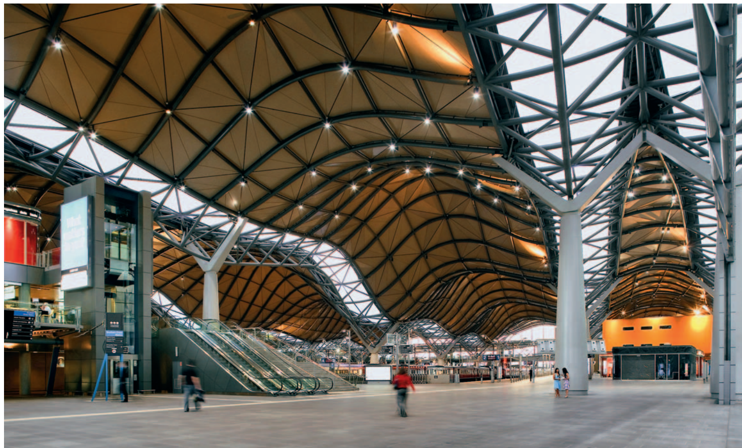
Nickolas Grimshaw. Southern Cross Station, Melbourne, 2007
