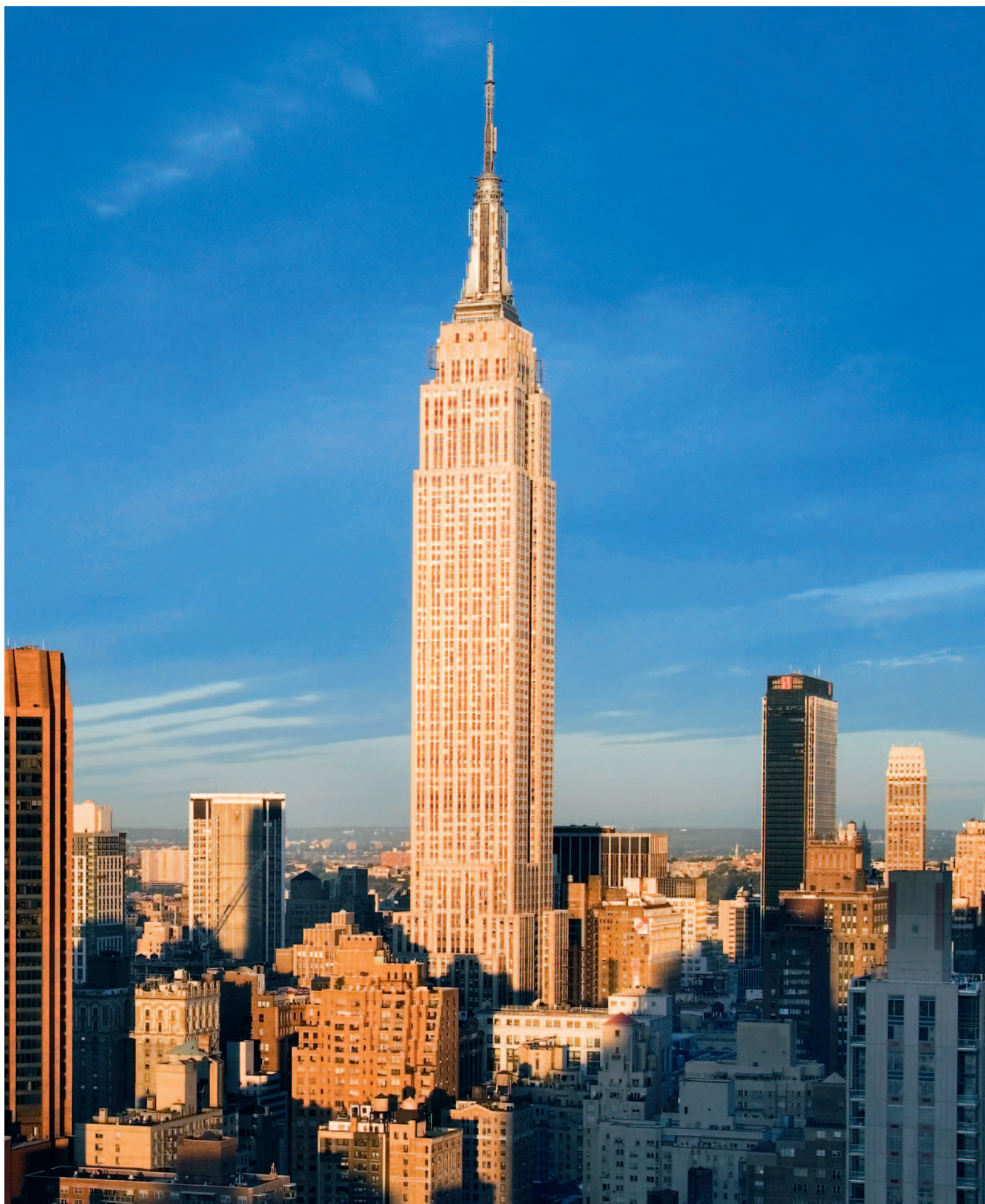
Gregory Johnson (Shreve, Lamb & Harmon Architects). Empire State Building, Manhattan, New York, USA, 1931 (house frame and window frames are made of aluminium)
