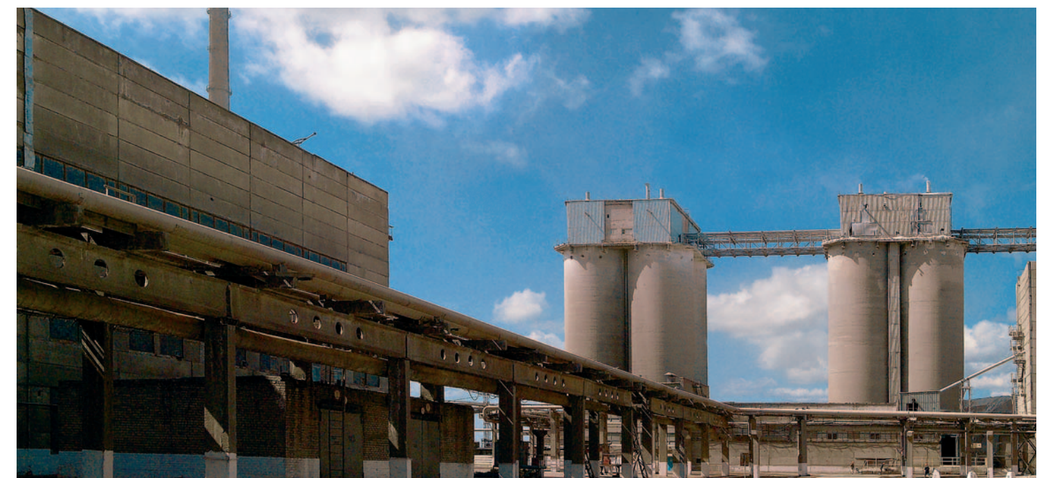
Achinsk Alumina Refinery
