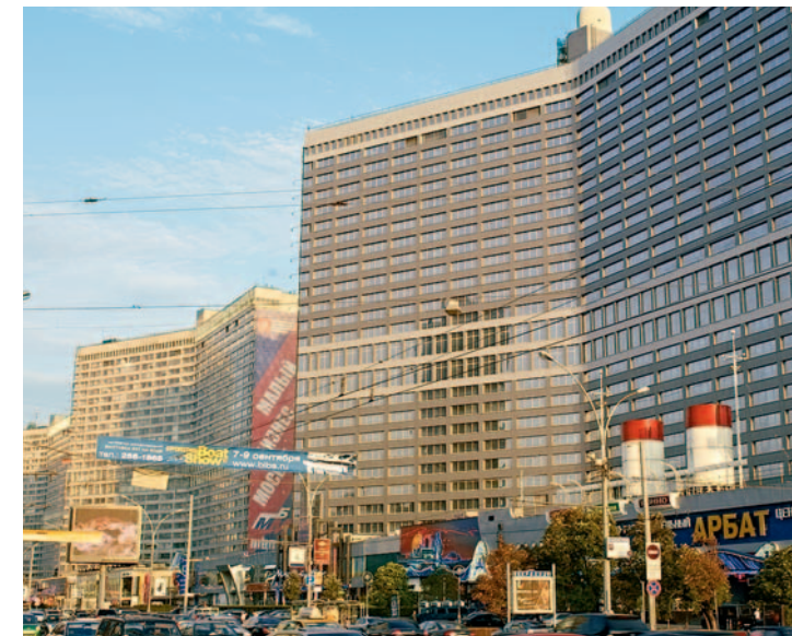
M.V. Posokhin. “Book” buildings Moscow, 1967 (stained-glass windows, doors and friezes of the interior are made of aluminium)
