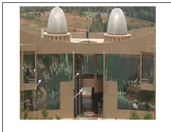
Figure-11: Front View of ISSDC Building
