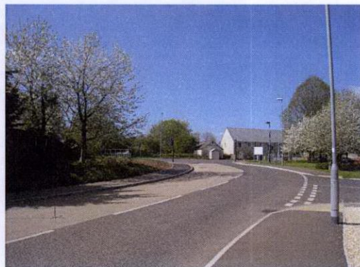
Wells Road access into Cobblers Way
