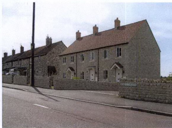
New cottages in Westfield, the original dwellings to the left of the photo
