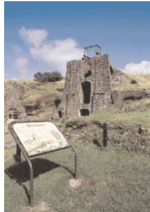
Interpretation panel at Blaenavon Ironworks ©Cadw
