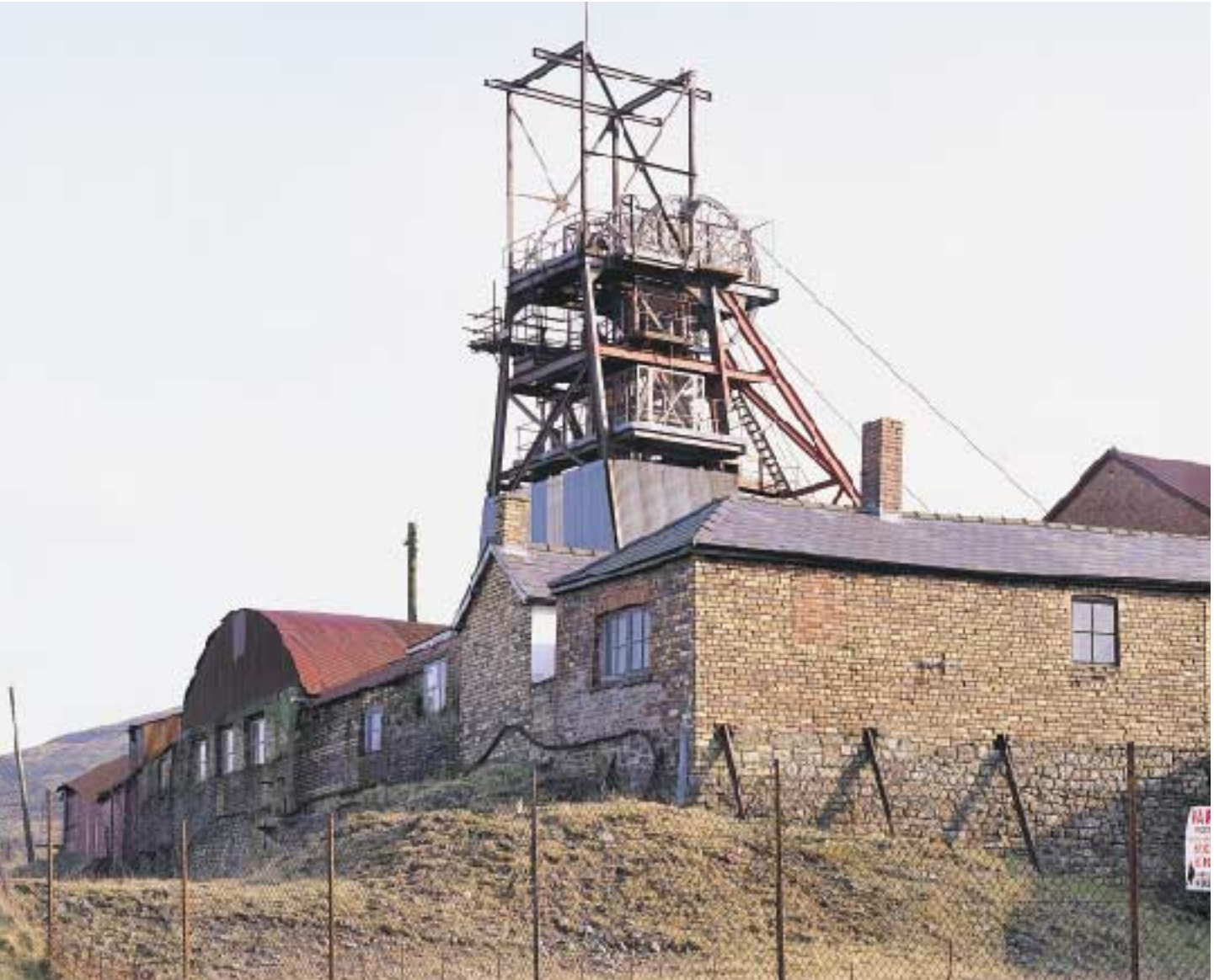
Big Pit Mining Museum, pit head winding gear ©Crown Copyright: RCAHMMW
