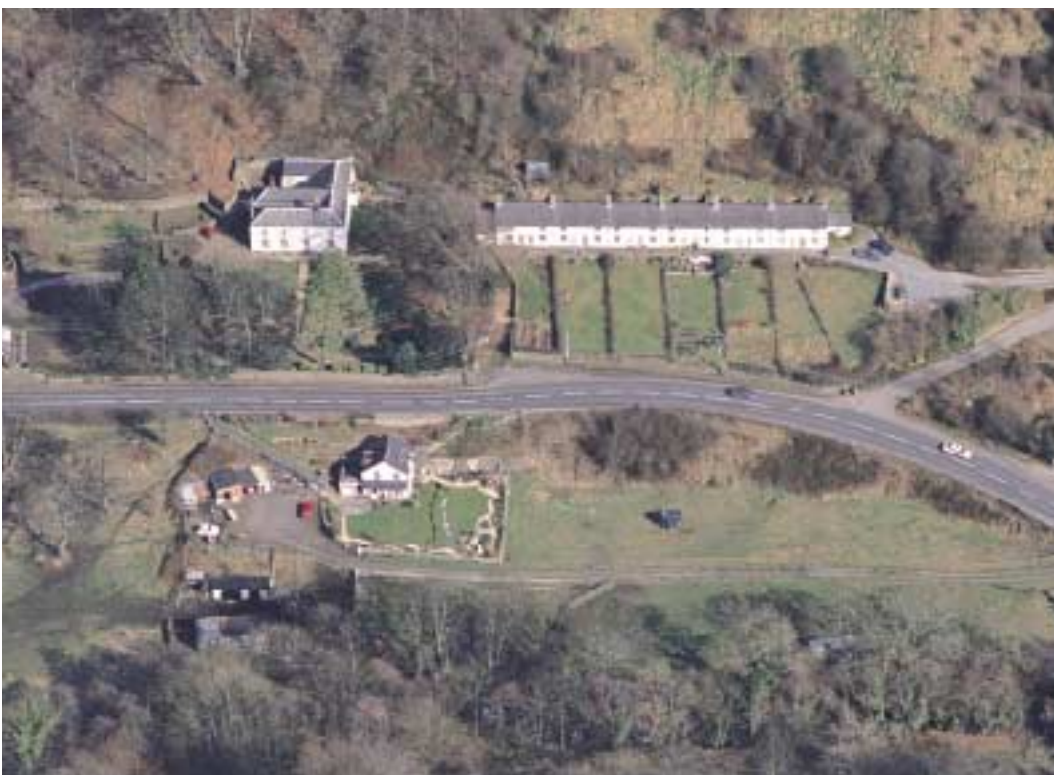
Aerial view of Cwmavon House and Forge Row (right). The site of Varteg/Cwmavon Forge is just below the main road, opposite Forge Row ©Crown Copyright: RCAHMW
