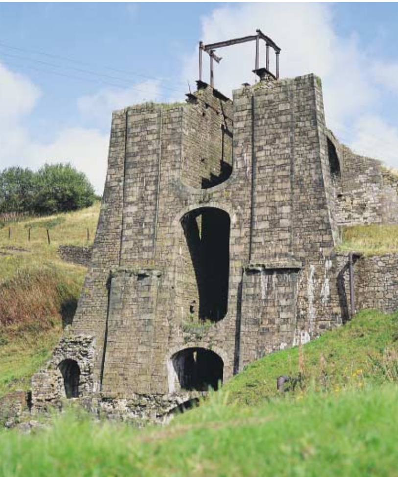
James Ashwell's water balance tower; a hydraulic lift built in 1839 ©Cadw
