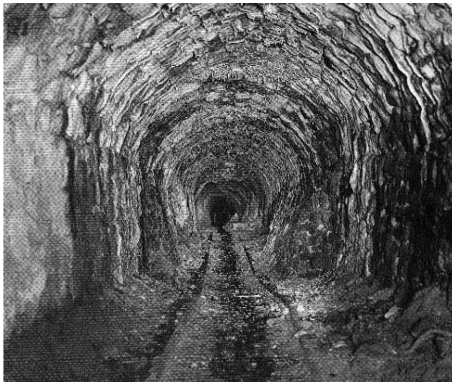
Engine Pit Level of 1810 still survives below Big Pit. The coal was turned into coke as one of the essential raw materials in the ironmaking process ©Crown Copyright: RCAHMW
