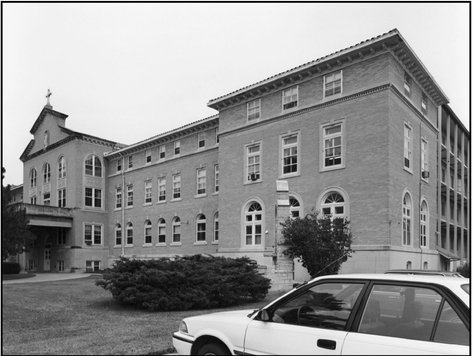
Photo 1 of 2—North façade looking southeast. Photo by Kent Behrens, 1994, Omaha City Planning Department.
