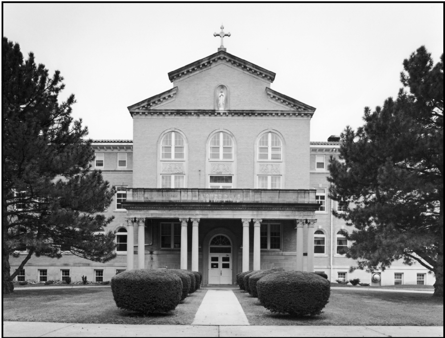
Photo 1 of 2—North façade looking south. Photo by Kent Behrens, 1994, Omaha City Planning Department.
