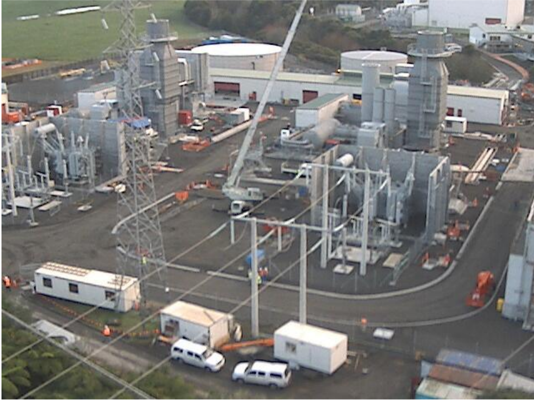
Photograph 1 Stratford Peaker Plant under construction, 1 July 2010
