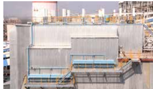
Hybridisation of all ESP's with bag filters, Vedanta Limited – Jharsuguda
