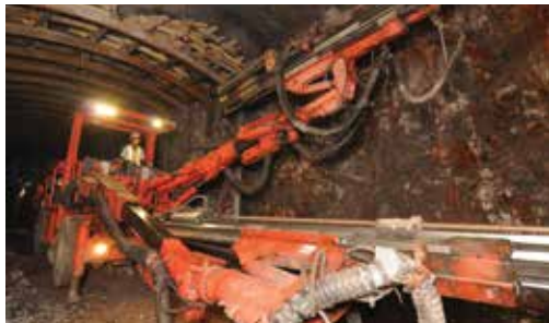
Excavation at Sindesar Khurd mine, HZL
