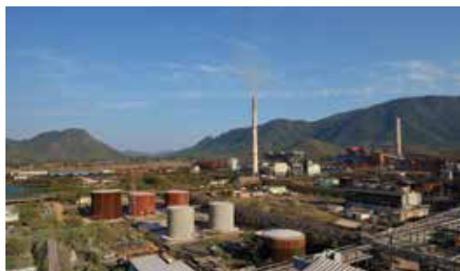
Panoramic view of the Lanjigarh Plant
