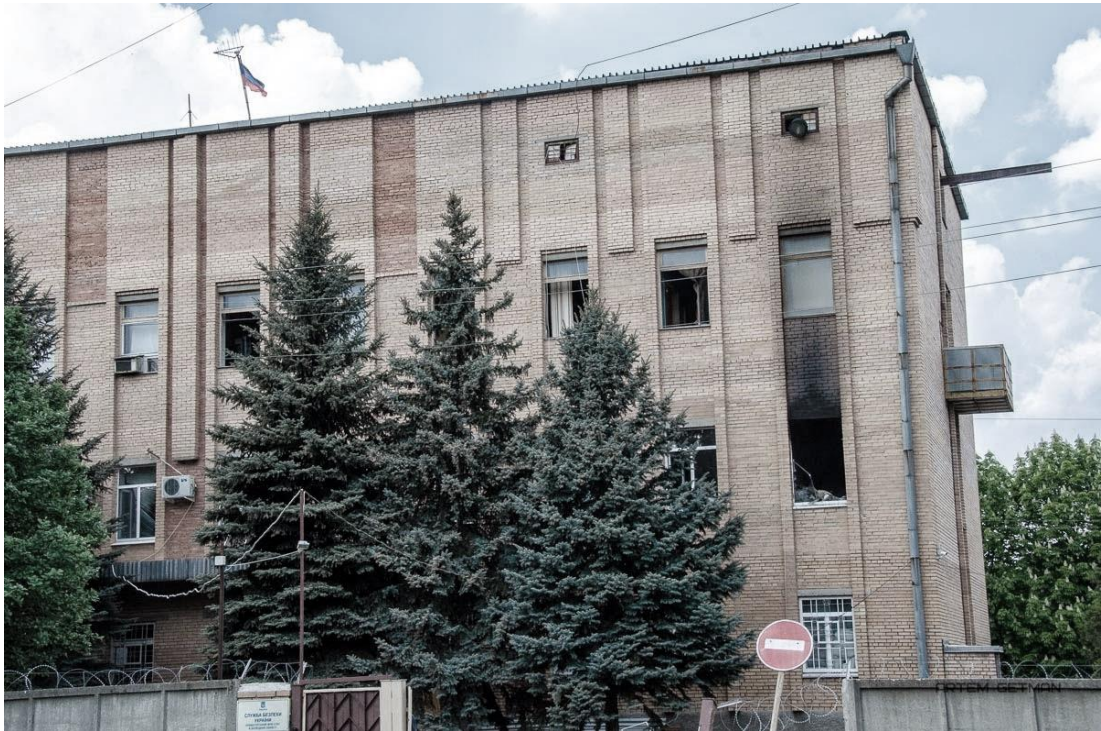
Building of the Security Service of Ukraine in Kramatorsk [41, 141]
