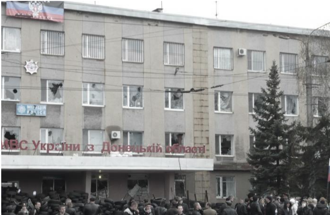
The building of a police station in Horlivka [131]
