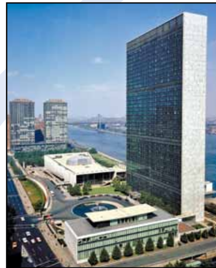
Same view of the site chosen for UN Headquarters, taken from Tudor City at 41st street, looking north to 48th street (left). United Nations Headquarters building in New York City as it stands today (above).
