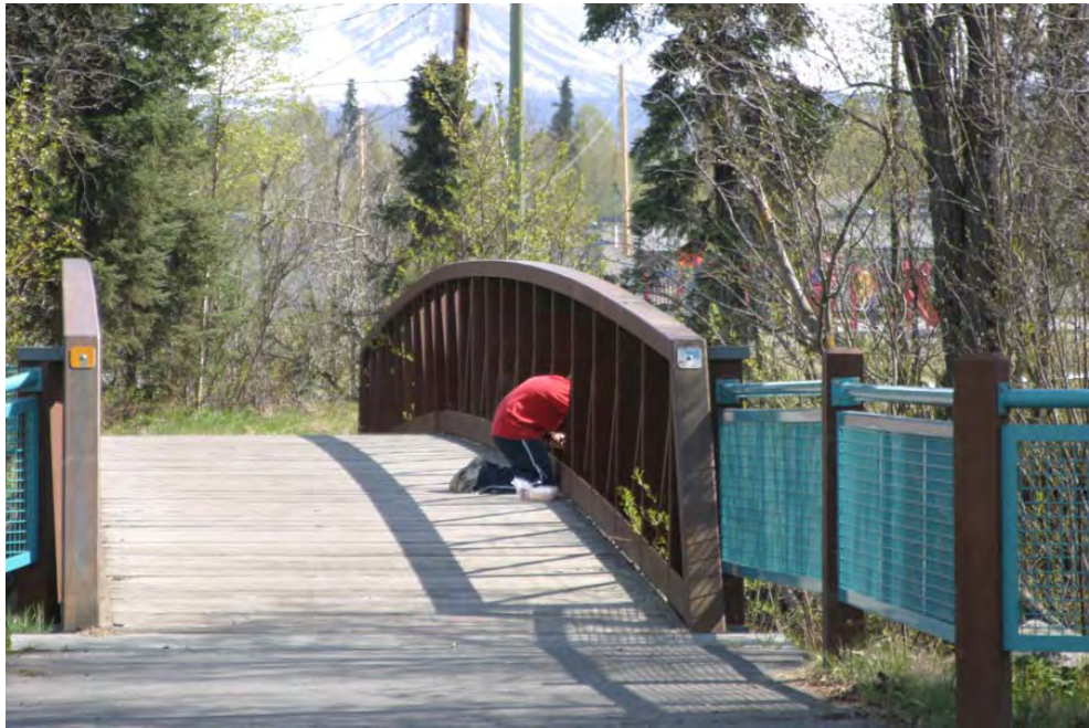
Fig. 58 – Campbell Creek bridge at Bancroft Greenbelt (photo by author)
