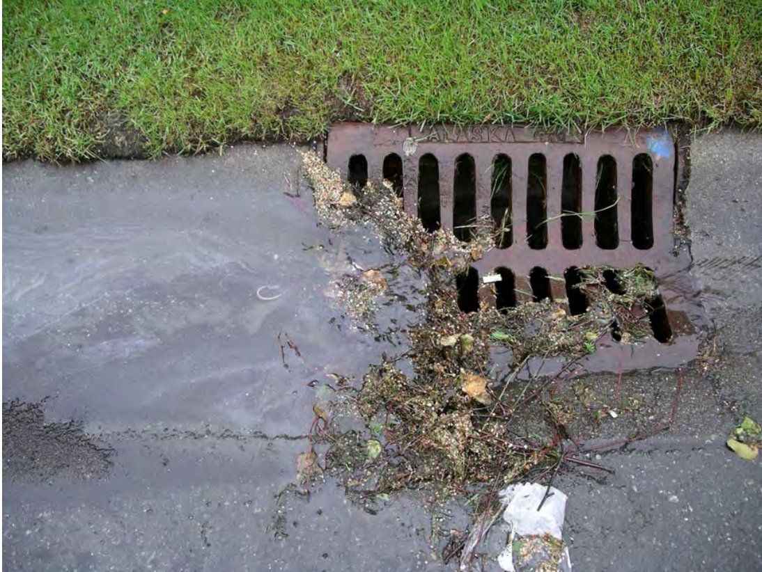
Fig. 79 - Storm drain that runs about 500' directly into Campbell Creek by the New Seward (photo by author)
