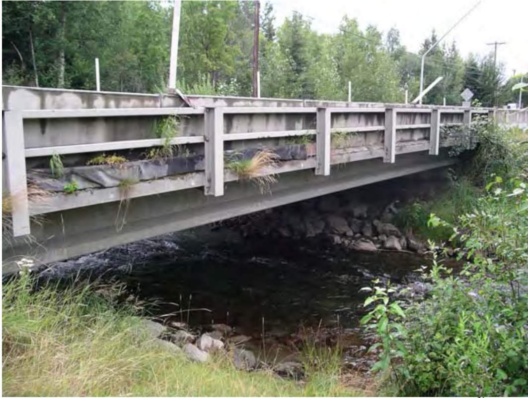
Fig. 34 - Potter/Dowling Bridge, August 2006 from south bank (photo by author) 31
