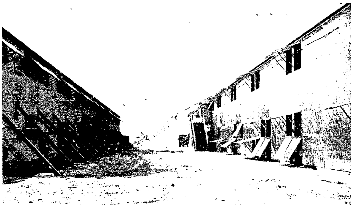
Figure 55. Buildings on Parry Island braced and with open windows in preparation for HARDTACK, OAK.
