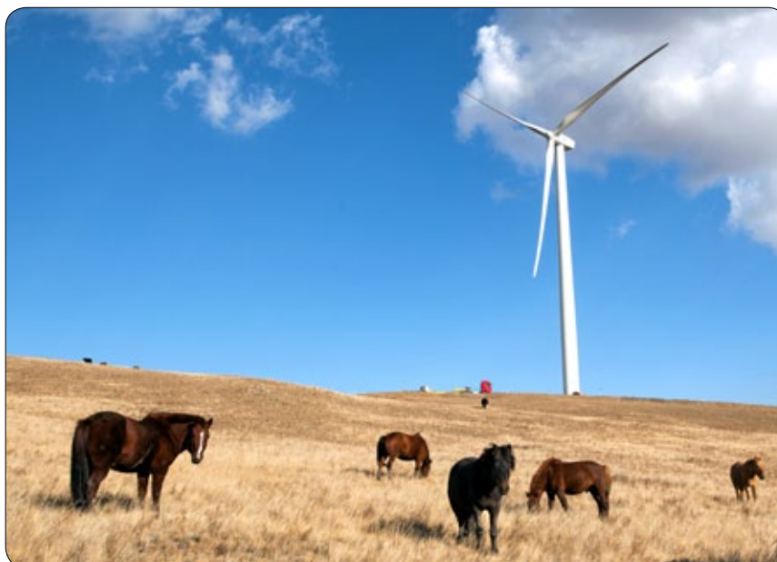
Finished in 2013, Salkhit will provide 5 per cent of Mongolia's electricity
