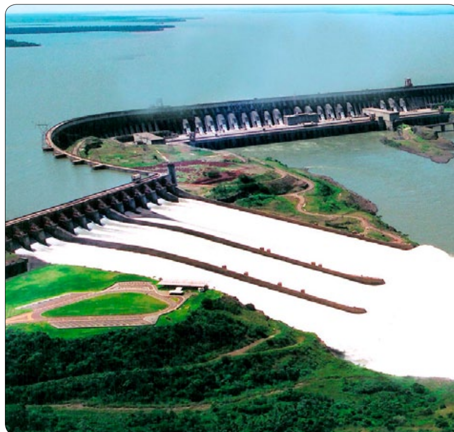
Half of Latin America's electricity is hydroelectricity
