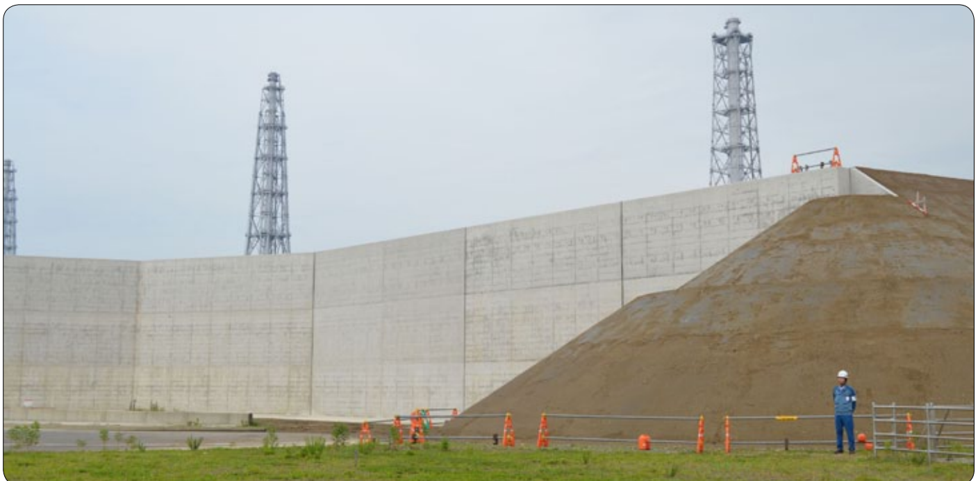
Flood barrier wall at Unit 1 of Kashiwazaki-Kiriwa Nuclear Power Station
