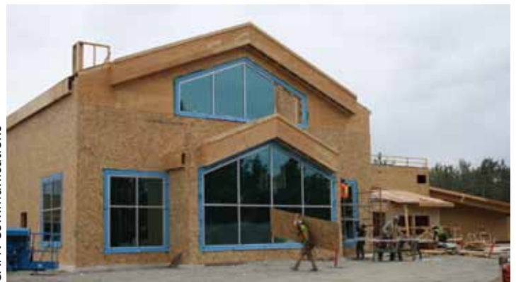
The busy Dä Kų Cultural Centre construction site - July 29, 2011.
