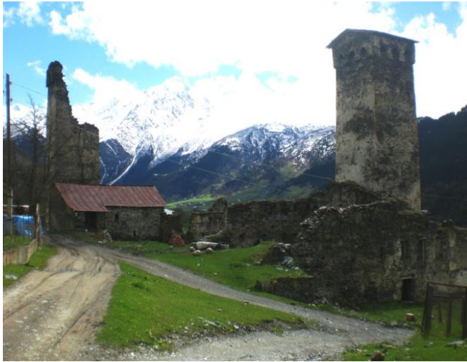
Photo 5.5.4. Tower selected for restoration (left) and tower in good conditions (right)
