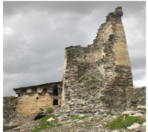
Photo 5.5.3. General view of the tower selected for restoration in village Zhamushi
