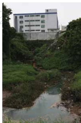
A hidden discharge outfall outside the Industrial Area
