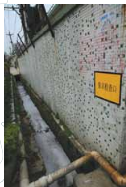
A discharge outfall of the facility
